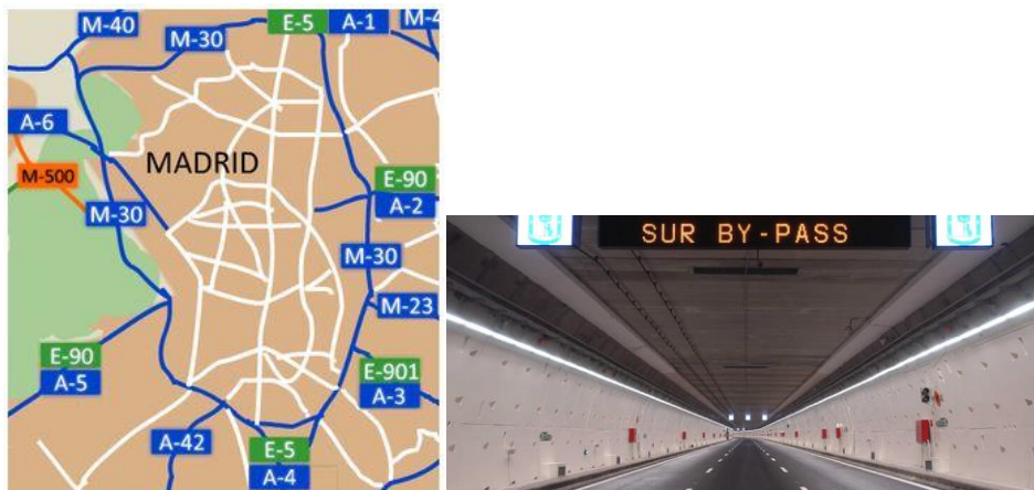
Figure 6: M30 route and tunnel picture
